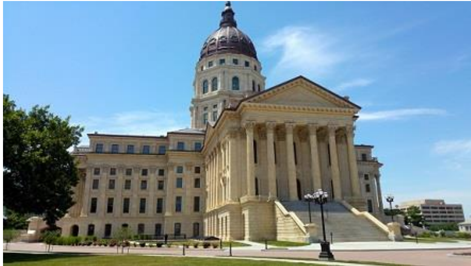
Kansas State Capitol Building
